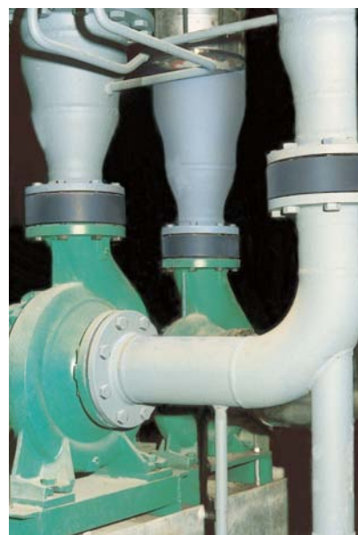
STENFLEX® type GRV at pumps in a heating system
