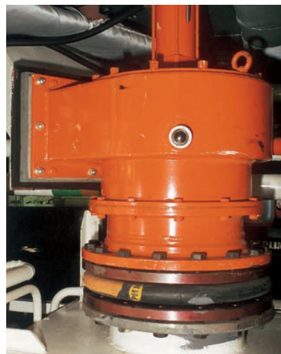
STENFLEX® type B-1 for compensating large movements
