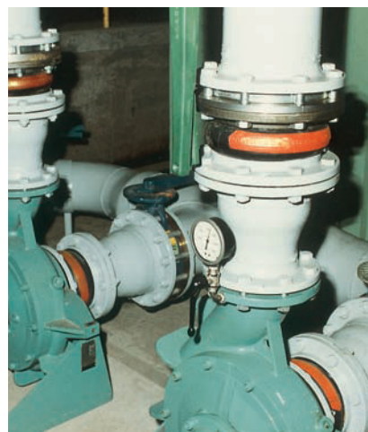
STENFLEX® type A-1 used at pumps
